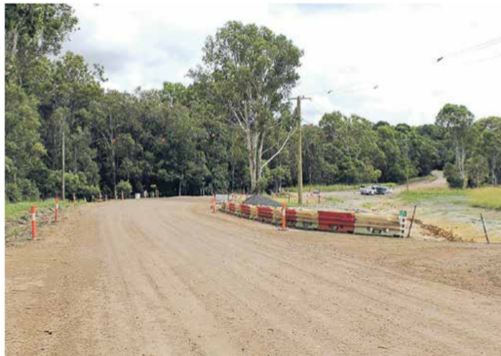
Doonan Bridge Road widening works. Photo: Richard Bruinsma
