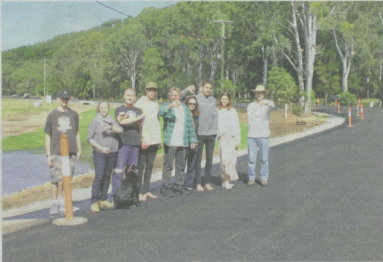
THUMBS DOWN: Residents are not happy with a corner on Doonan Bridge Rd.
